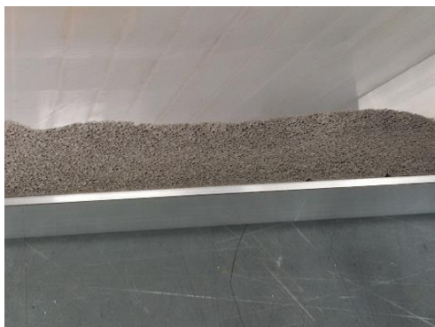
Figure 35 Expanding sealant tape right after application
